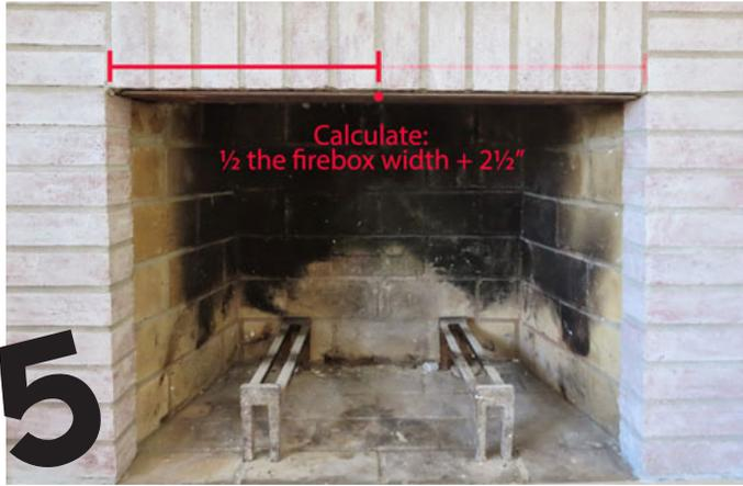
5 Calculate 1/2 the width of your firebox + 2.5 inches. This is the length that you need to cut your rods. Make sure NOT to cut them on the end with the screw hole. Use a hacksaw to cut them. Example  $21'' + 2.5'' = 23.5''$
