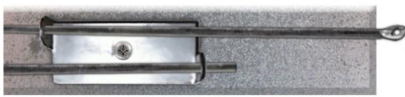
How the rods are threaded through the mounting bracket that is attached to the center of the lintel iron.
