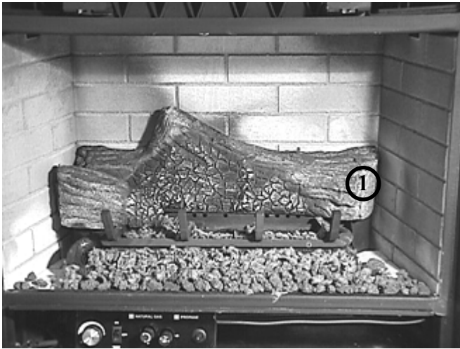
Place the rear log in the center and against the brick at the rear of the firebox.
