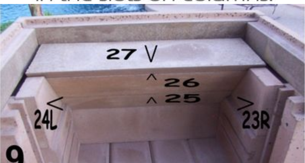
9. Place L. and R. upper blocks as shown. Place 2 back angle blocks as shown. Place top cover. (Except on open fireplace.)
