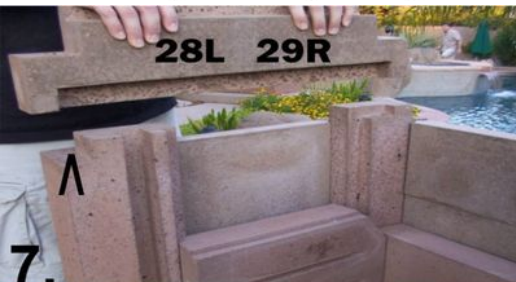
7. Place left and right cap blocks in the slots on columns.
