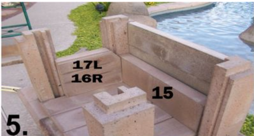
5. Place the back, left and right fire chamber blocks. (except on open fireplace.)
