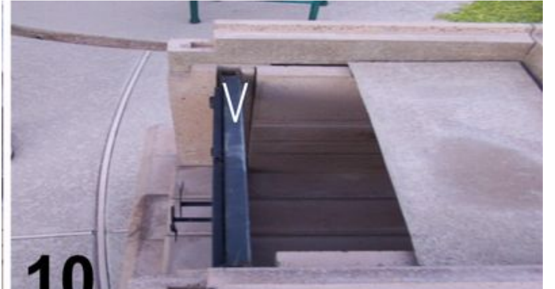
10. Slide door assembly down into front columns. Place front cap block in slots on side block cap's.
