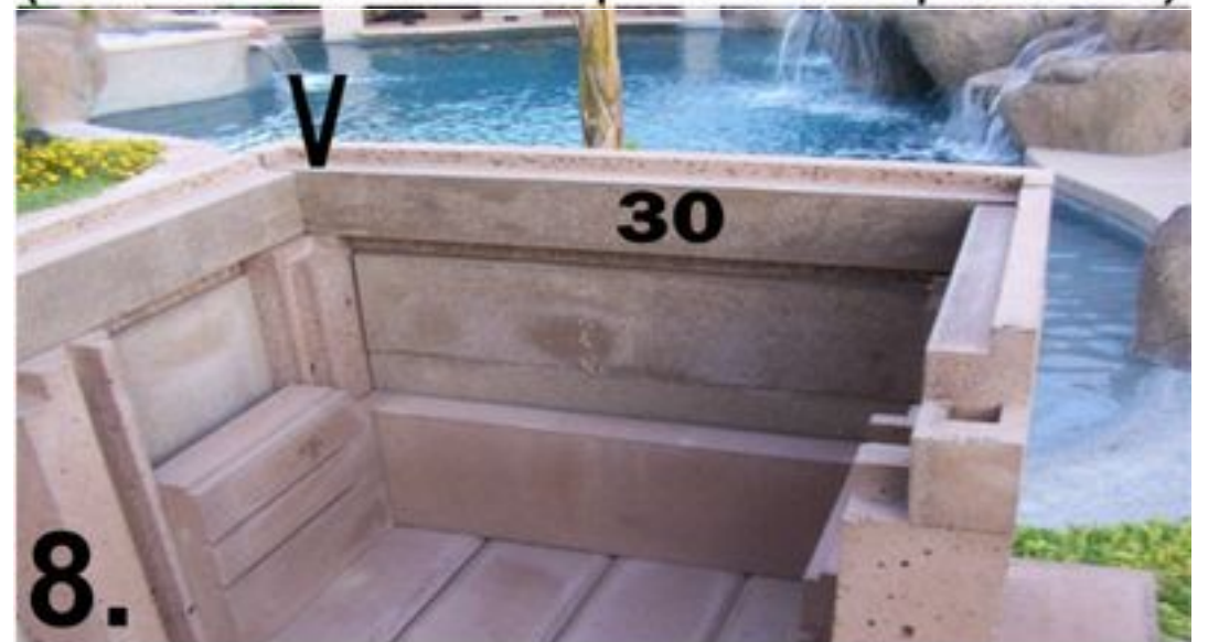
8. Place rear cap block in slots on side cap's.
