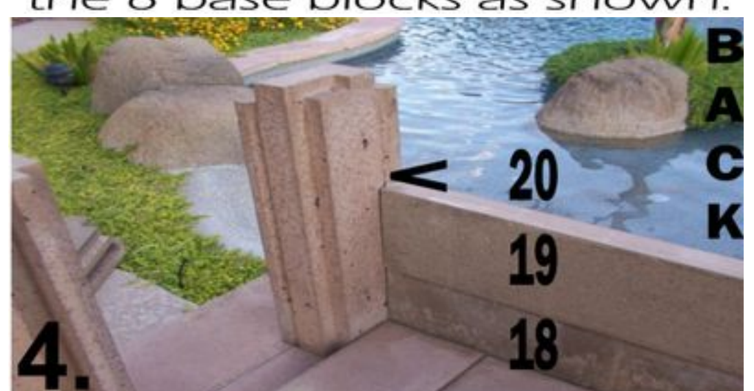
4. Slide down 3 back blocks in v-groove. (Use back screen on open fireplace.)
