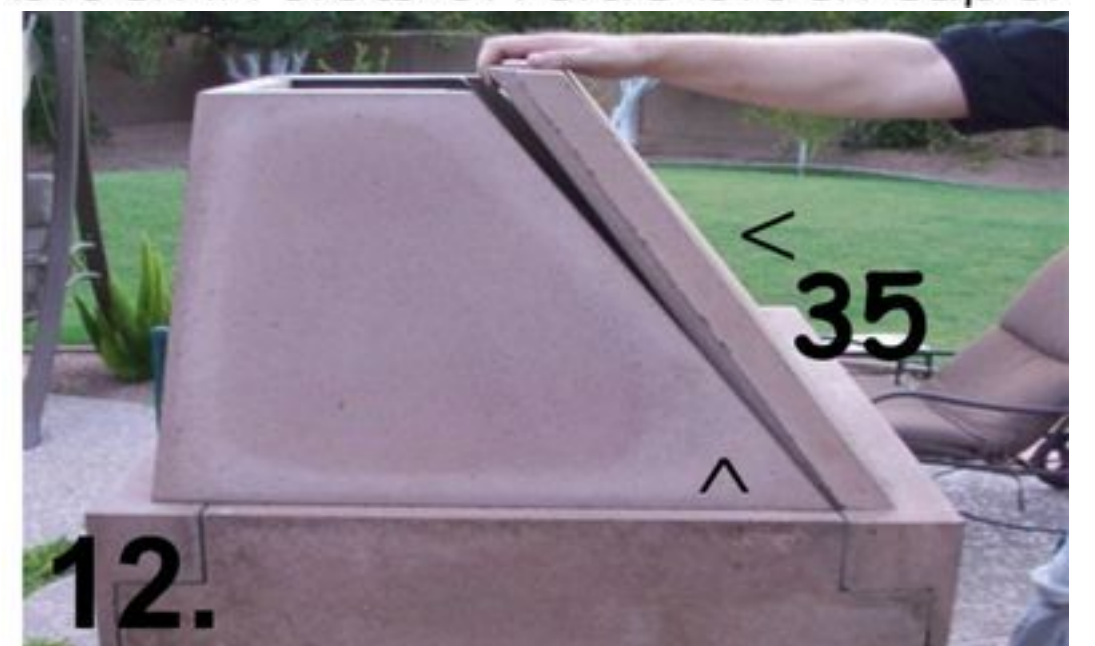
12. BE PATIENT! Set one end of the front panel into position. Lift the front of the opposite side panel until the panels line up. Gently lower both panels and lean face block back. Watch your fingers.
