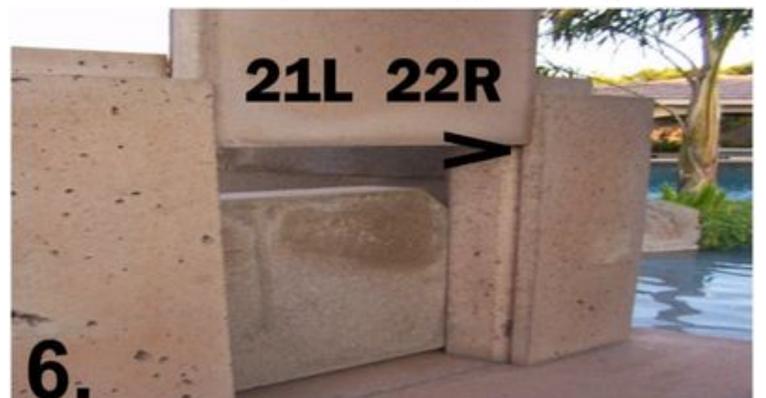
6. Slide left and right side panels down in v-groove. (Screens for open fireplace.)
