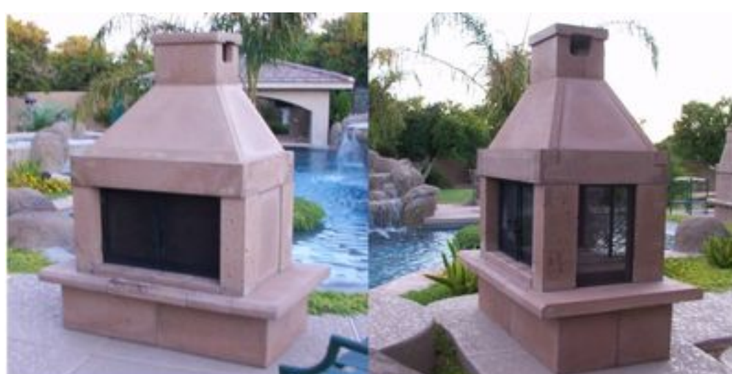
Place 2 chimney blocks and top block. Assembly complete.
