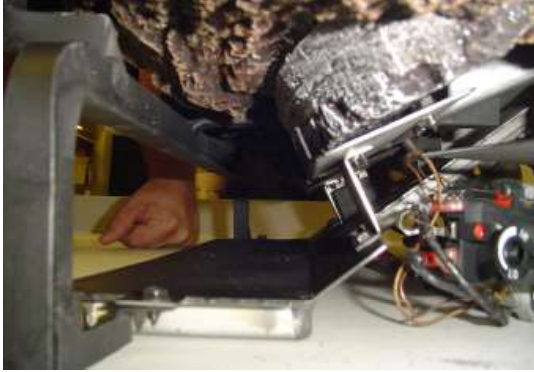
Figure 24C - Installing Right Front Log, Side View
