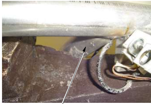
Vertical Portion of Burner Tube
