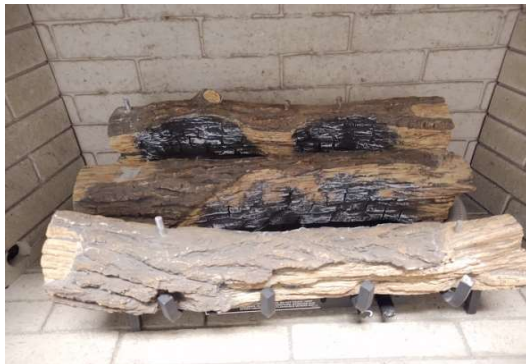
Figure T - Install Front Log
