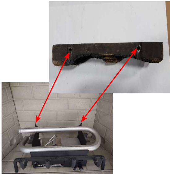
Figure N - Rear Log Placement
