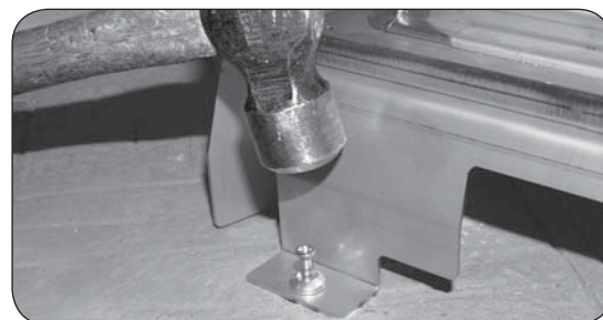
Fig. 15-3 Install hammer screws
