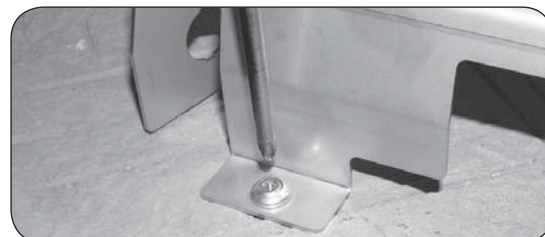
Fig. 15-2 Fasten hammer screws
