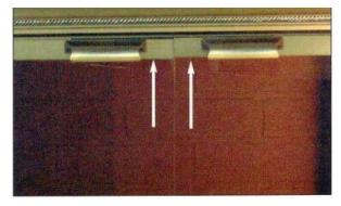
STEP 13 Check alignment of door panels.
