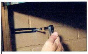
STEP 9 Install 1/4" X 1 1/2" lag bolt and lock washer into the anchor using a 7/16" wrench.
