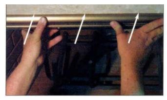
STEP 6 Press top of door frame tight against opening of fireplace. Inside mount align depth.
