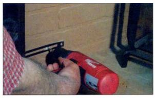
STEP 10 Drill 5/16" hole in center of mounting straps slots. Repeat steps 9 & 10 but do not tighten lag bolts.
