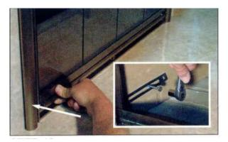
STEP 12 Move bottom of door in or out to align face of doors. Gently open doors, and tighten bottom lag bolts and lock washers. Close and recheck alignment.
