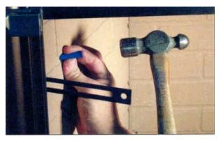
STEP 8 Bend mounting bracket back out of the way, insert anchor and tap with hammer until flush. Return bracket to its original position.
