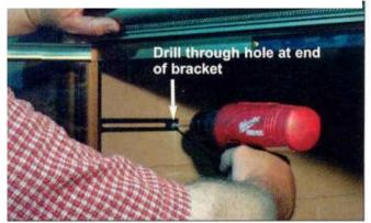
STEP 7 Using a 5/16" masonry bit, drill holes at the end of mounting brackets. Press at top of frame while drilling. NOTE: For metal fireboxes, do not use lead anchors, use #8 x 1" TEK screws.
