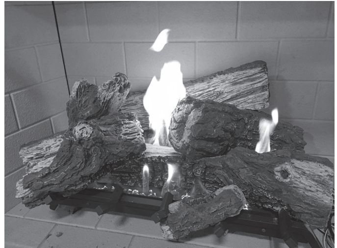
Figure 6.13 - Correct Appearance of Rear Flames
