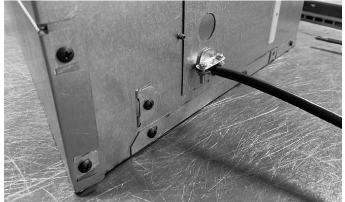
Figure 5.2 Reattaching Junction Box Cover
