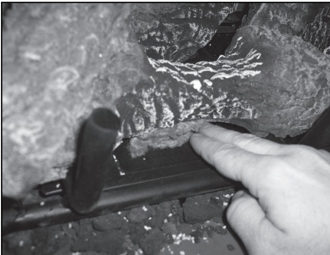
Figure 14.24 Placement of Rockwool Under Front Logs
