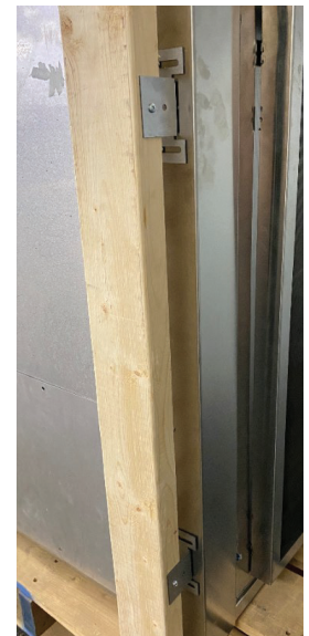
Figure 6.8 Fasten installation brackets to wall framing
