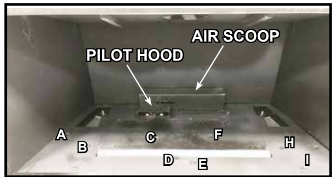
Figure 2. Empty Firebox with Shoulder Screw Locations
