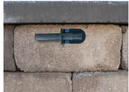
Figure 6.6 – Fasten down the bracket
