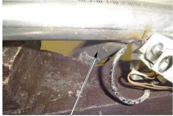
Vertical Portion of Burner Tube
