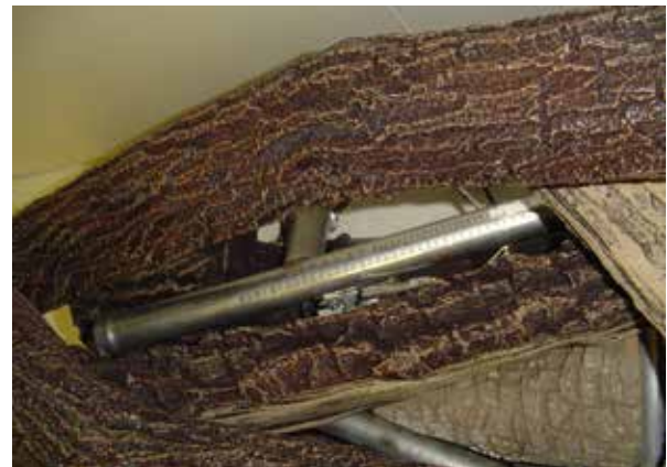
Figure 25A - Installing Back Top Log, Top View
