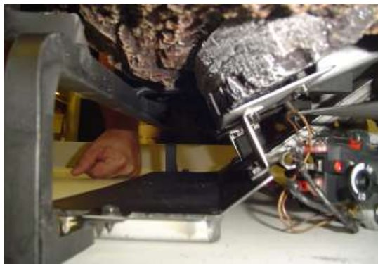
Figure 22C - Installing Right Front Log, Side View
