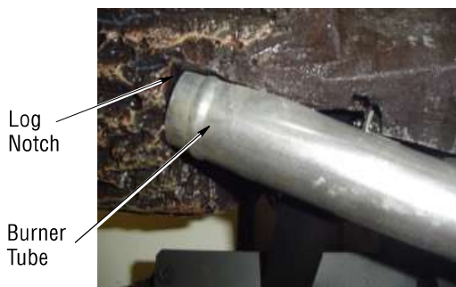
Figure 23A - Installing Back Left Log
