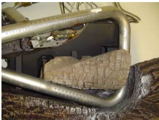
Figure 25A - Installing Charred Log Top View
