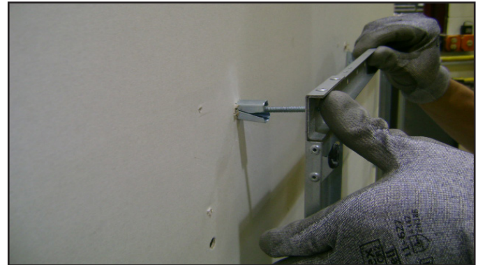
Figure 29. Installing Anchors in Hollow Wall
