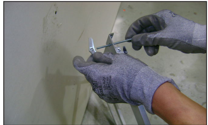
Figure 28. Toggle Bolt Installation through Mounting Bracket
