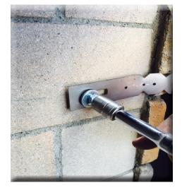
**6.** Tighten lag bolt (provided ) until flange is snug. Adjust as needed to make door fit well on opening face.
