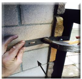
**4.** Hammer or bend tab to tightly fit to fireplace opening. With a marker or pencil. Mark within slot for the lead anchor placement.
