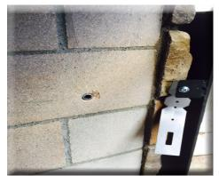
5. Drill hole with a 5/16" into firebrick or 3/8" drill bit. (not provided). Insert lead anchor.
