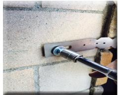
6. Tighten lag bolt (provided ) until flange is snug. Adjust as needed to make door fit well on opening face.
