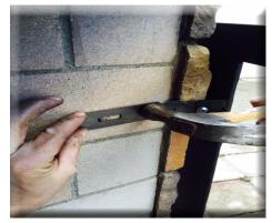
4. Hammer or bend tab to tightly fit to fireplace opening. With a marker or pencil. Mark within slot for the lead anchor placement.
