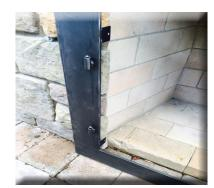
1. Place door frame against opening to find which set of install tabs are best suited for your installation. The tabs should protrude into the fireplace opening.
