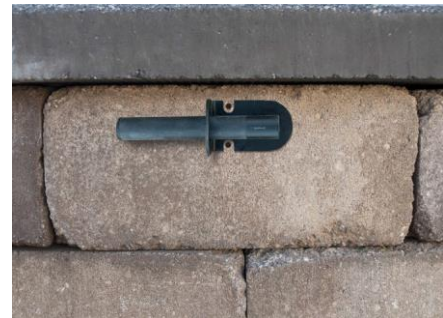
Figure 6.4 – Dry fit the bracket
