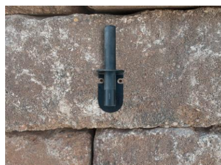
Figure 6.8 – Dry fit the bracket
