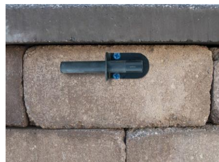
Figure 6.5 – Fasten down the bracket
