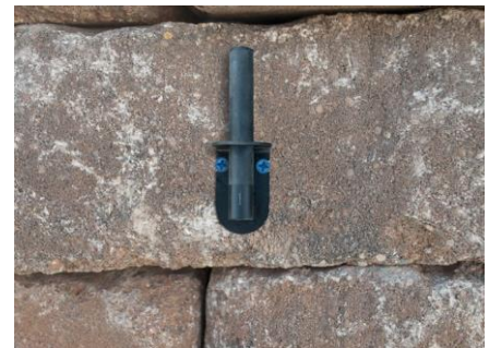
Figure 6.9 – Fasten down the bracket
