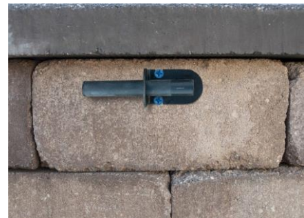
Figure 6.5 – Fasten down the bracket
