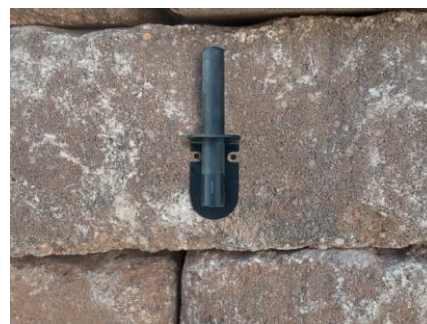
Figure 6.8 – Dry fit the bracket
