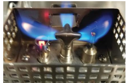
Figure 9.2 – Pilot flame coverage of thermocouple.
