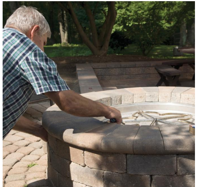
Figure 9.1 – Match-Lit test start-up
