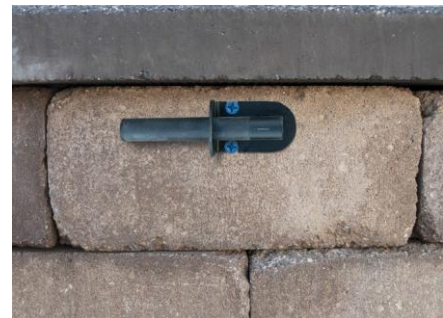
Figure 6.6 – Fasten down the bracket
