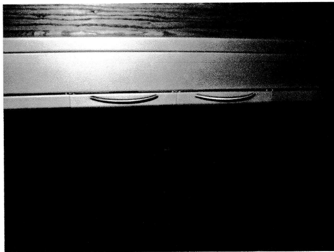
PROPERLY ALIGNED BIFOLDS
