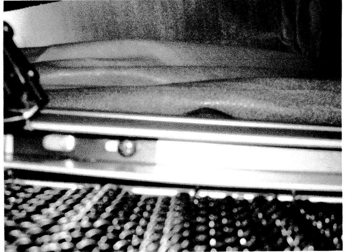
Step 8 Slightly loosen screws and adjust hinges so that bifolds are level at center and tighten screws
