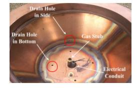
Apply pipe dope/tape to the gas stub and thread the AWEIS Ignition Control Box onto the gas riser as shown in the photo at right.
