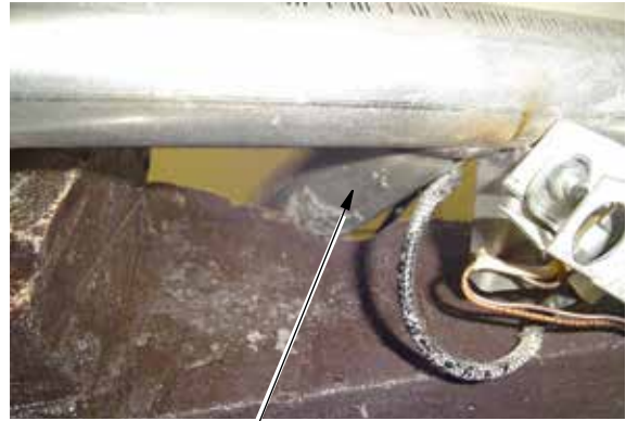
Vertical Portion of Burner Tube
