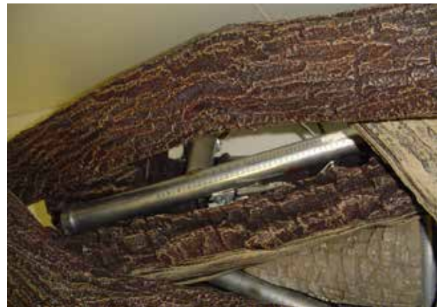
Figure 25A - Installing Back Top Log, Top View
